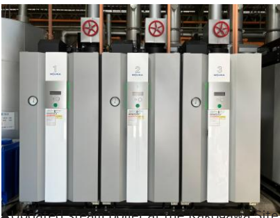
Replaced steam boiler at the Kakogawa Site
