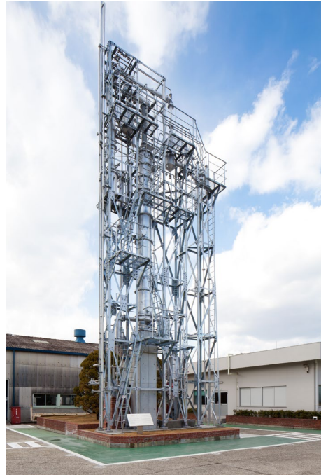
Pilot Plant (Relocated in 2012)
