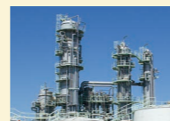
Present tall oil distillation plant
